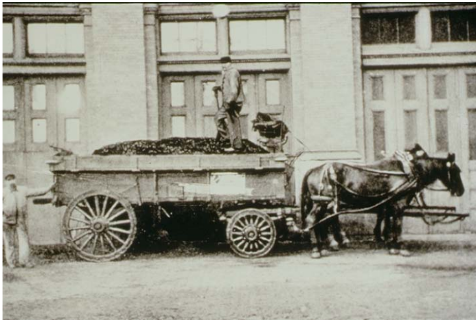
Figure 1-2: Bottom ash "cinders" from We Energies' Wells Street Power Plant destined for road surfacing and other applications.
