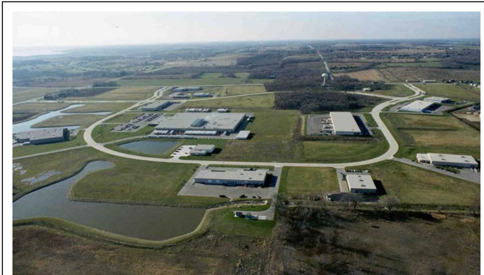
Figure 4-19 : Aerial view of the village of Sussex Corporate Center that was paved with high-volume fly ash concrete.
