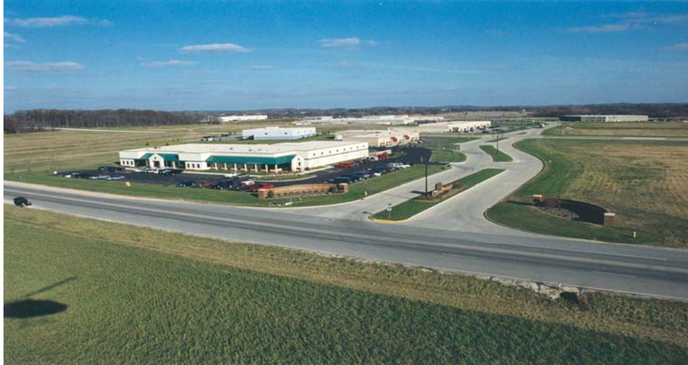
Figure 4-18: Sussex Corporate Center boulevard entrance paved with high-volume fly ash concrete
