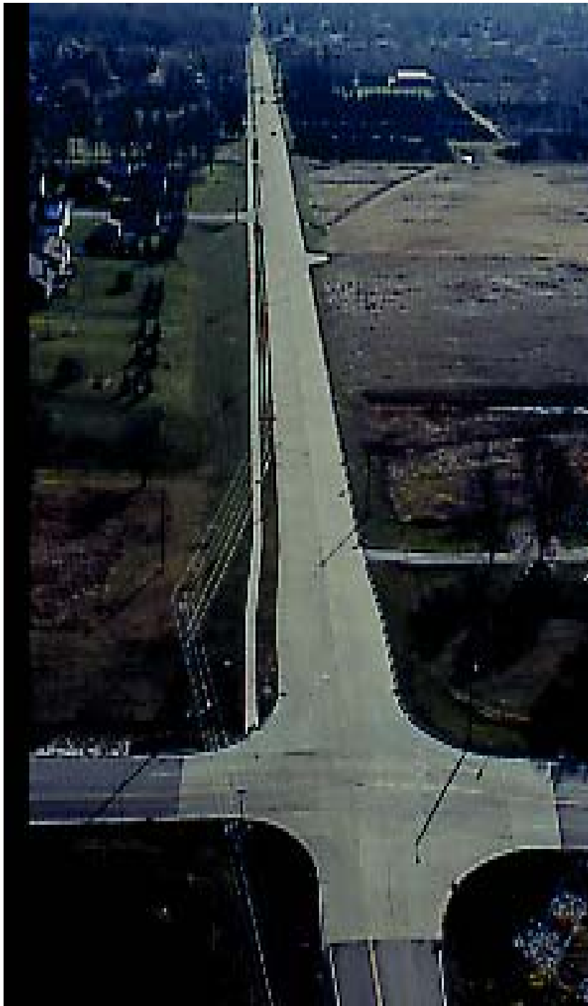
Figure 4-21: Another view of Maple Avenue located in the village of Sussex paved with high-volume fly ash concrete.
