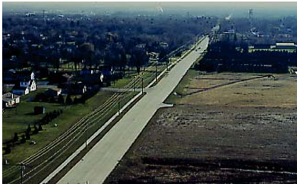
Figure 4-20 : Maple Avenue roadway and sidewalk located in the village of Sussex and paved with high-volume fly ash concrete.
