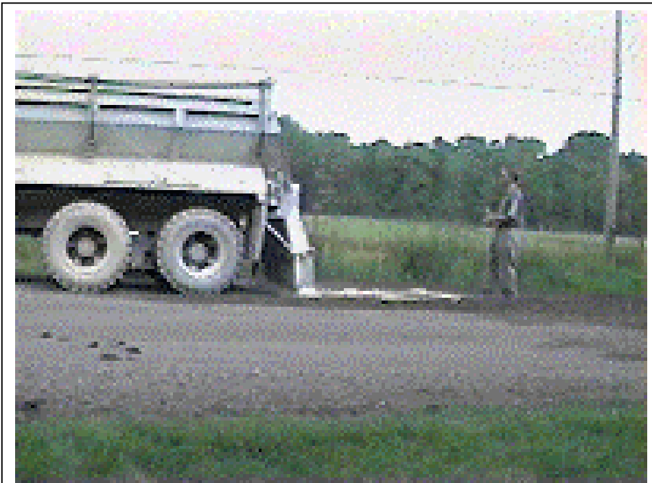
Figure 7-2: Fly ash being placed uniformly on the pulverized pavement.
