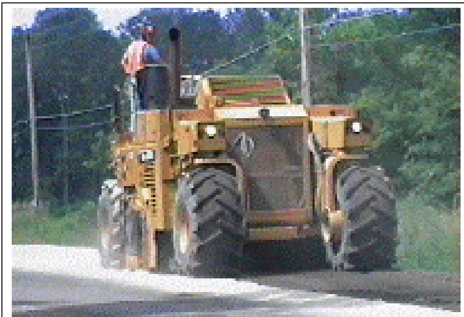
Figure 7-3: Pavement being repulverized after fly ash application.
